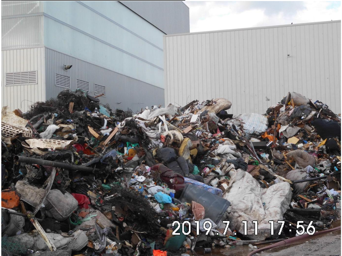
Photograph 5 Burnt waste, incinerator walls unaffected
